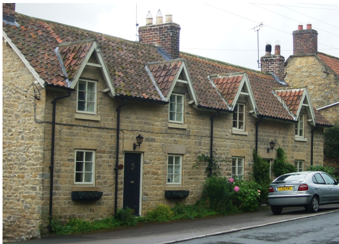
Swiss Cottages, Main Street: gabled half dormers typical of Oswaldkirk's paired Victorian cottages
