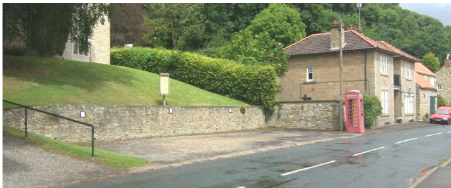
Loss of traditional boundaries and areas of hard standing can be detrimental to the street scene
