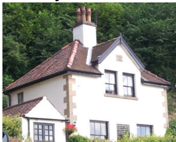
Crag Cottage, Main Street: central chimney stack
