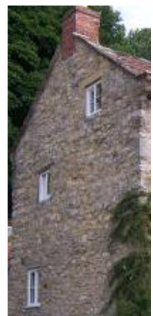
Random rubble stone gable to vernacular building
